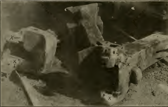
CRACKED DRAWBARS PREPARED FOR WELDING, VIRGINIAN RAILROAD.
